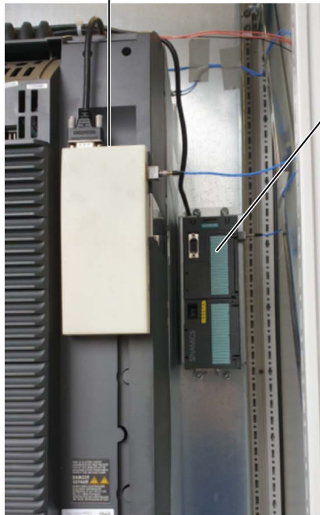
Figure 8-3 Control Unit Adapter Kit and separately installed Control Unit
