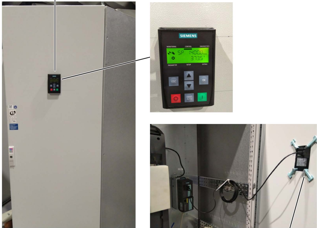
Figure 8-4 Control cabinet with installed operator panel
